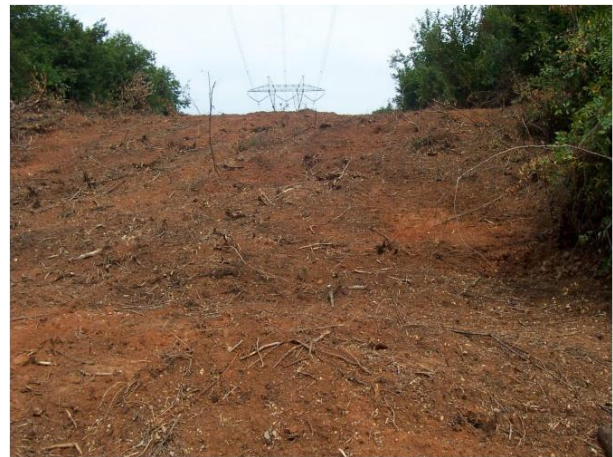
Fig. 3. Destruction of vegetation due to power lines
