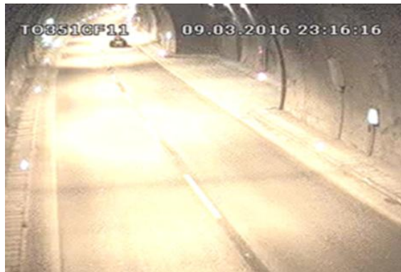
Fig. 7. Interior zone of tunnel
