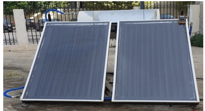
Fig. 2. Thermosiphon solar water heater.
